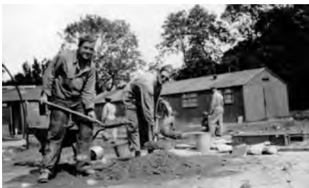
Eighth Air Force base construction was often accomplished without the heavy equipment we would expect to see today.
