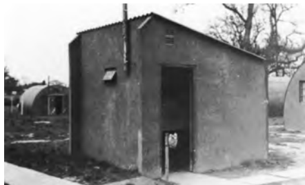
A Station 153 latrine. The Eighth Air Force air base project comprised one of the biggest civil engineering projects ever undertaken.
