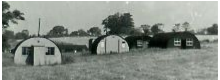
Postwar scene of the 412th site where 16-foot Nissen huts comprised five sergeants' quarters. Barely visible behind the middle hut is a latrine. In the background is a Thorne building, a wooden frame that was covered in bitumen-coated paper. This structure was one of five officers' quarters on the site. On the right side of the picture is a barracks hut. To the far right is the end of the cinema building.
